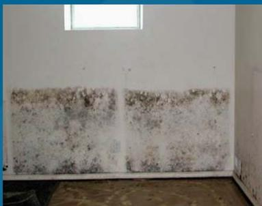
Basements and crawlspaces are often damp. The moldy walls in this picture are probably from rainwater that is not directed away from the house.
