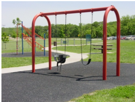
Poured in Place
