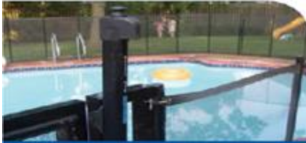
Barriers, Entrapment, and Electrical Safety
